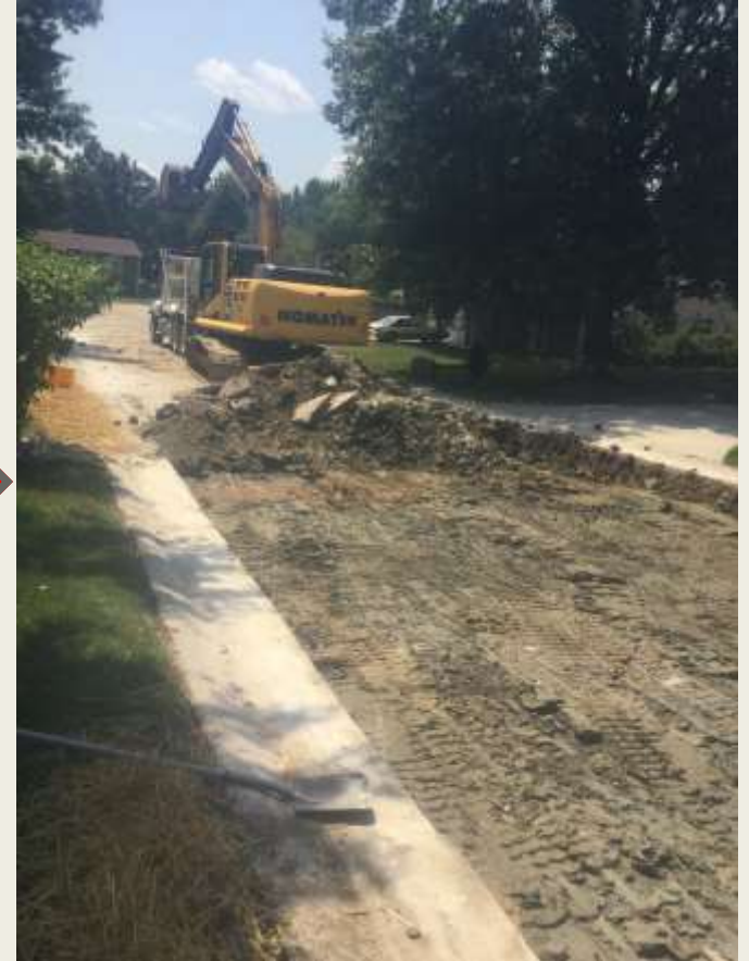
Step 3: Pavement Removal/Excavation
