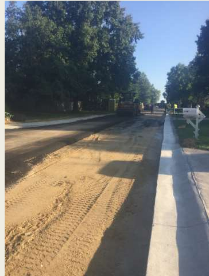
Step 5: Asphalt Paving
