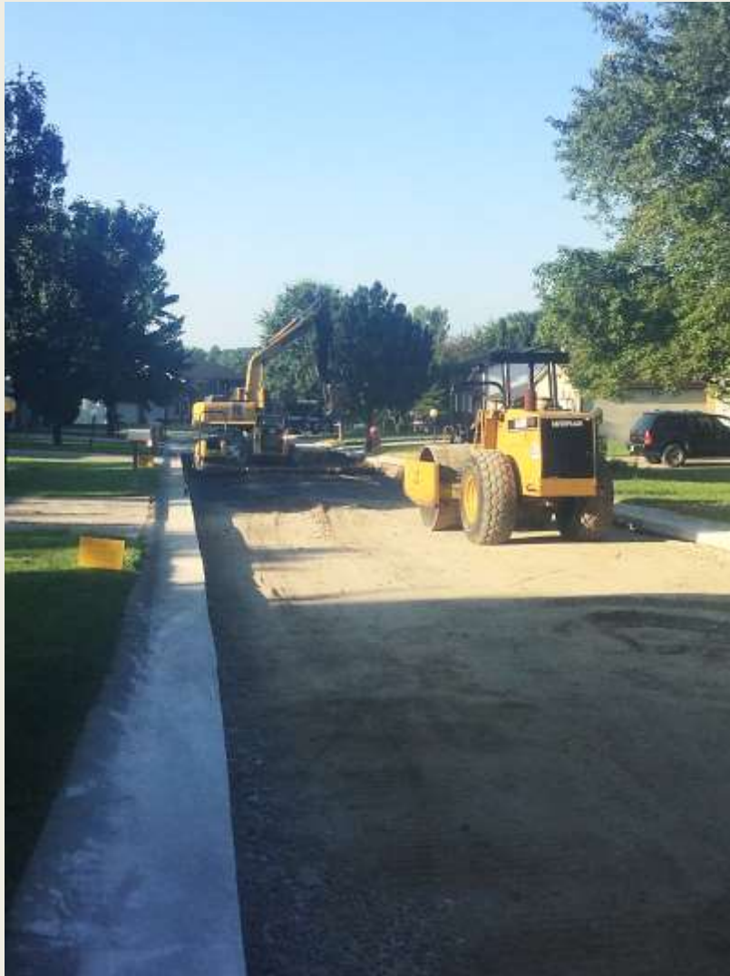
Step 4: Fabric & Base Rock Installation
