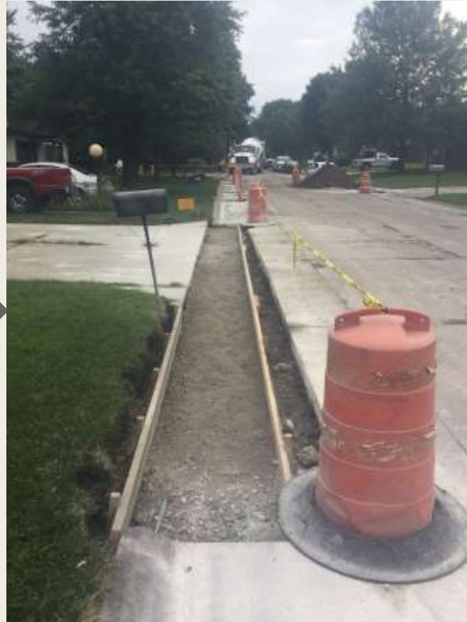
Step 2: Curb and Gutter Repair
