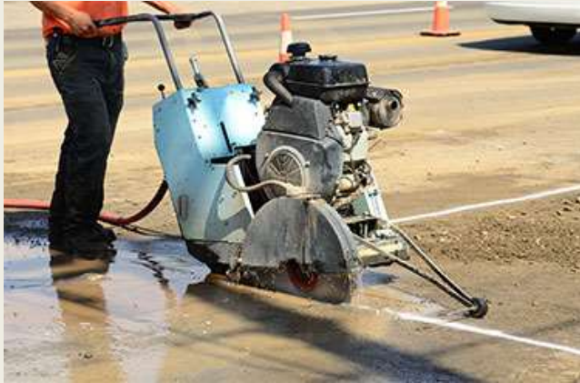
Step 1: Saw Cut Gutterlip
