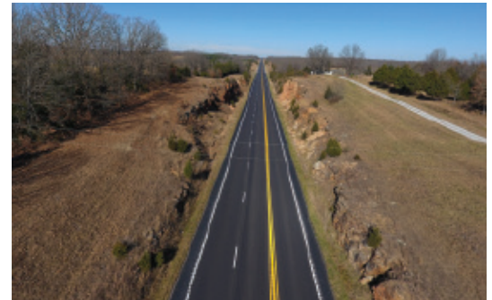
US 63 Pace Construction Co. Inc.
