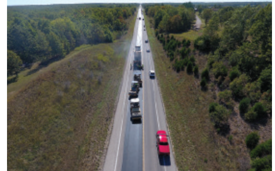
US. 63 Pace Construction Co. Inc.
